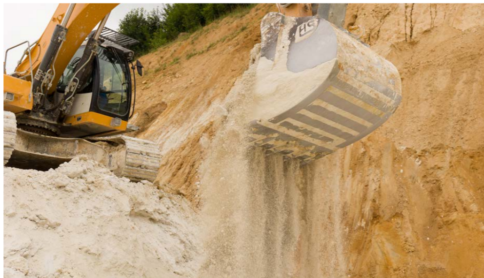
Excavation is carried out with state-of-the-art machinery
